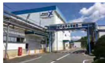
Nagase ChemteX's Fukuchiyama Plant
