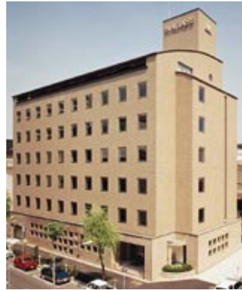
Nagoya Branch Office
