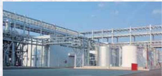
Chemical Recycling Plant within Sharp's "Green Front Sakai"
