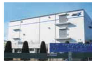
Harima Plant: New formulated epoxy resin production facility
