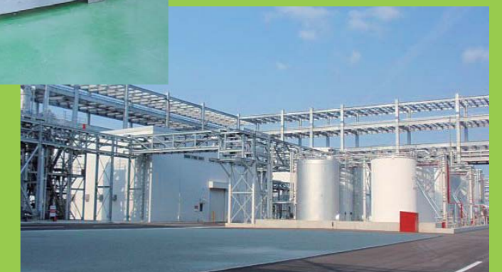
Chemical recycling plant within Sharp's “Green Front Sakai”
